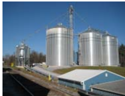
White Oak's 300,000 bushels of grain storage and new corn receiving and transfer system
